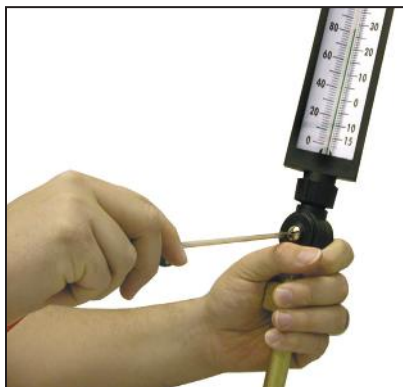
Loosen single screw (A).
